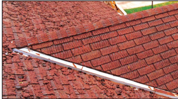
Hail damaged asphalt shingles.
