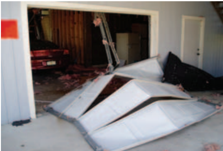
Garage door damage documented during the 2004 hurricane season.
